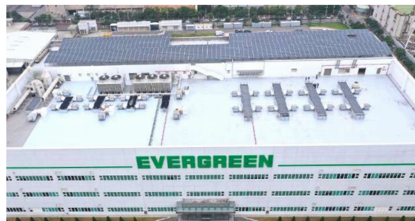
Solar photovoltaic system installed on the rooftop of the manufacturing business.
